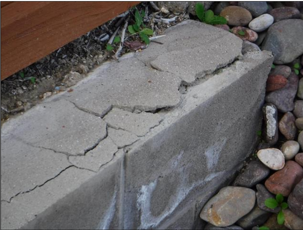
2.4 Item 1(Picture) Retaining wall efflorescence
