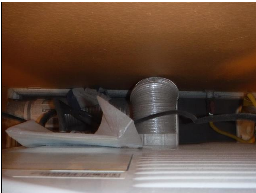
4.14 Item 2(Picture) Lint build up behind dryer
