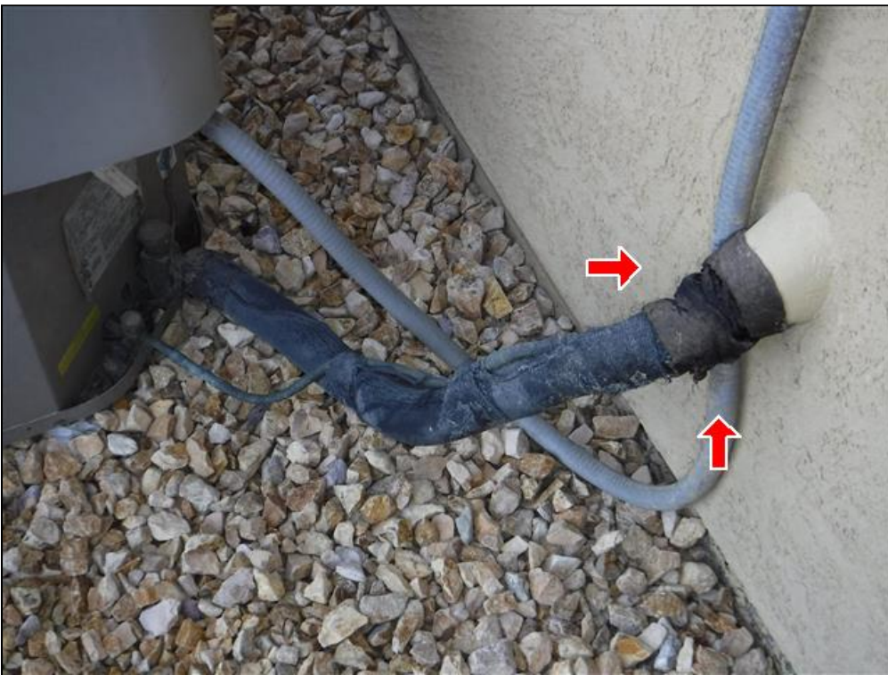
10.6 Item 2(Picture) Insulation on cooling line
