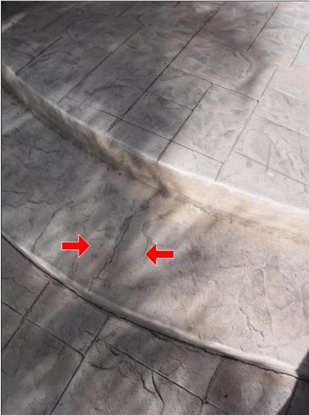
2.3 Item 1(Picture) Crack on front steps to house
