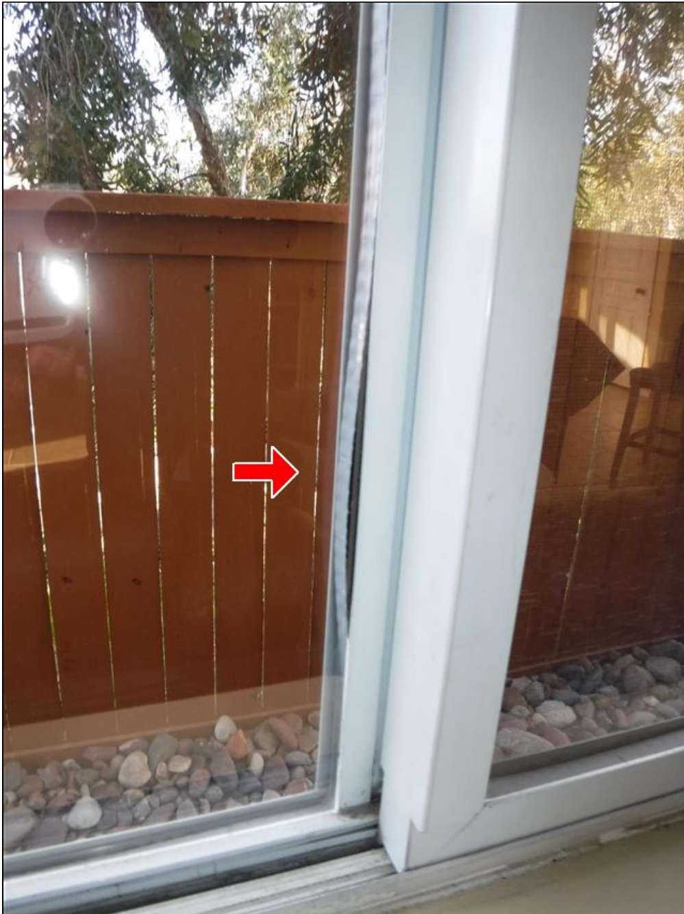
2.2 Item 3(Picture) Broken window seal
