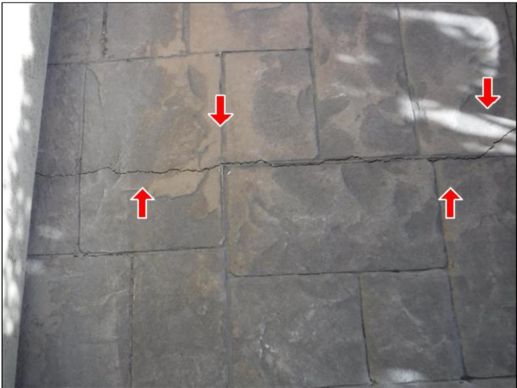
2.3 Item 3(Picture) Front stoop crack
