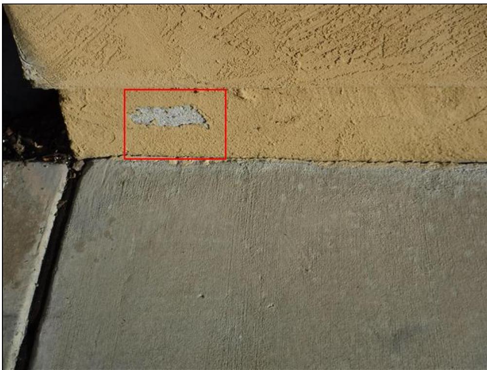
2.8 Item 2(Picture) Chipped paint on exterior slab
