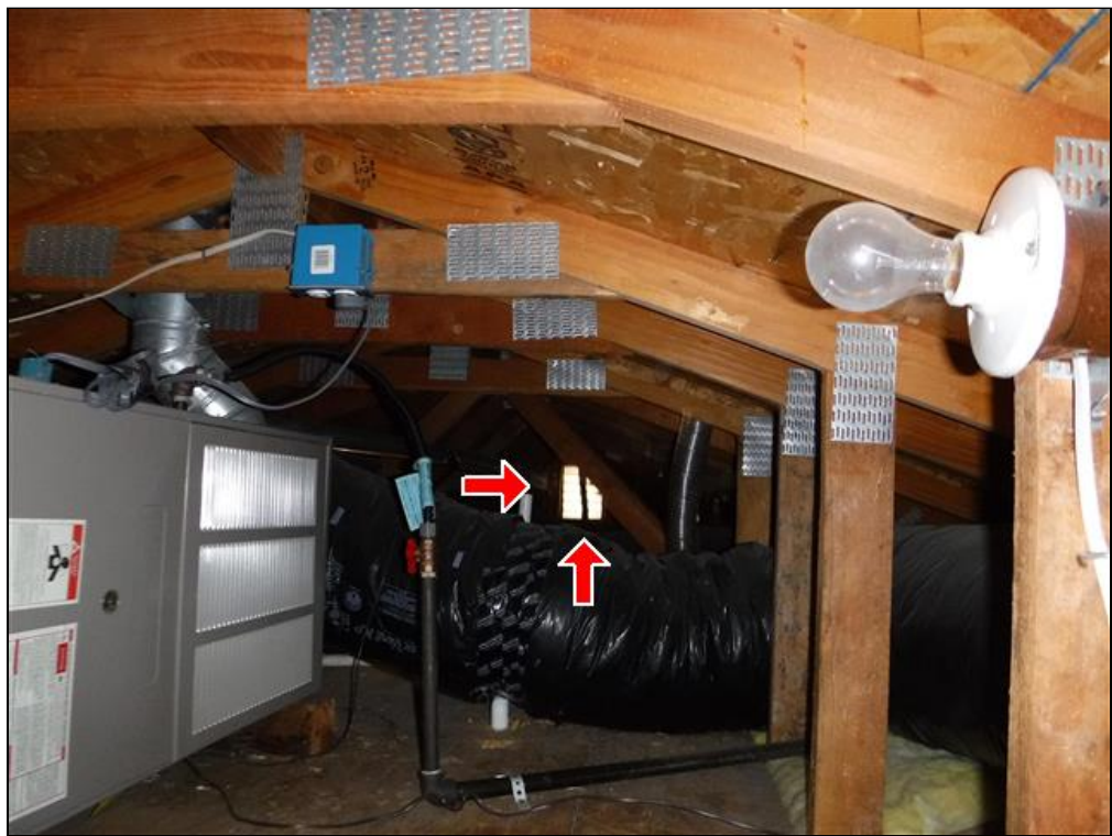
1.2 Item 1(Picture) Gable Vents in the attic
