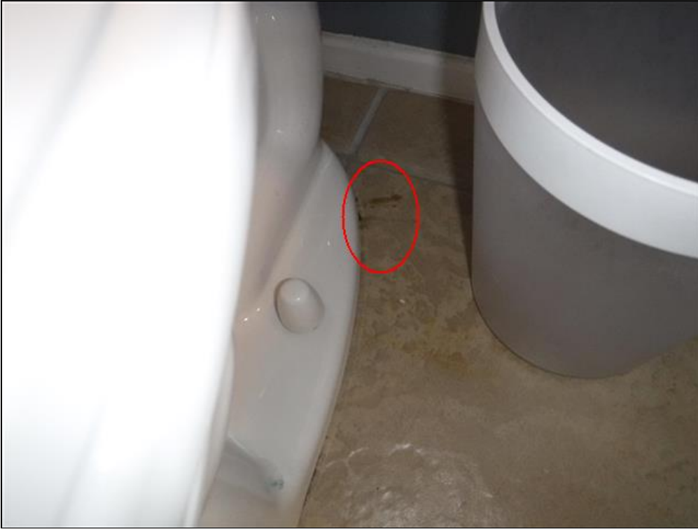
8.1 Item 1(Picture) Moisture at base of half bath toilet
