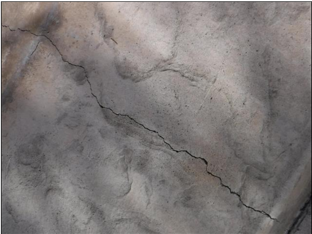
2.3 Item 2(Picture) Crack on the front stoop
