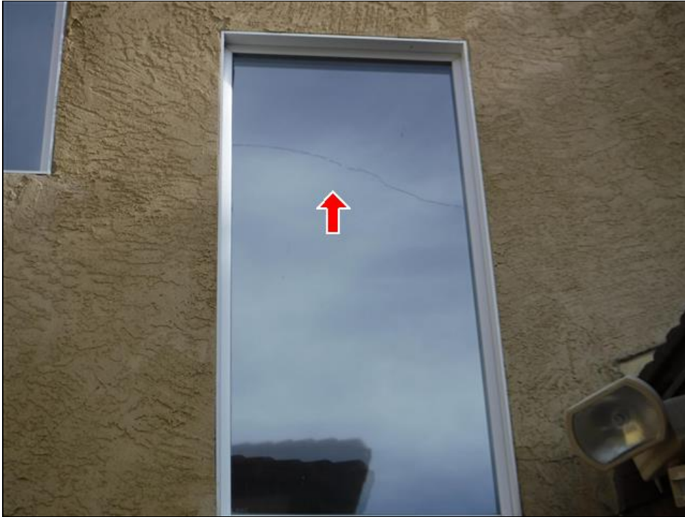
2.2 Item 1(Picture) Window tint bubbling
