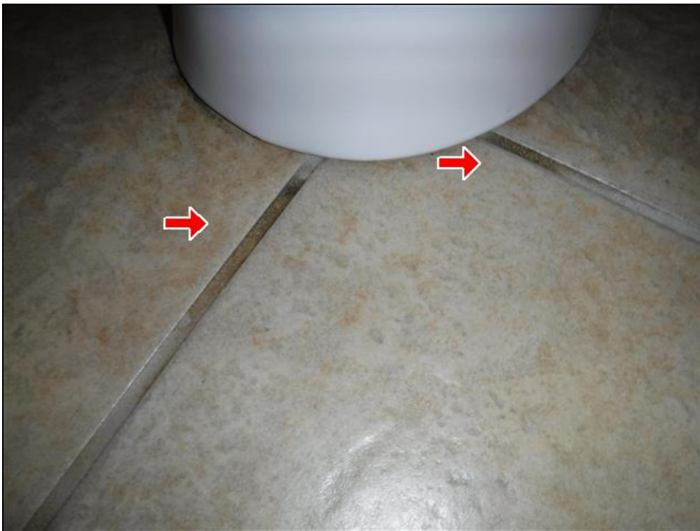
8.1 Item 2(Picture) Moisture stains in grout
